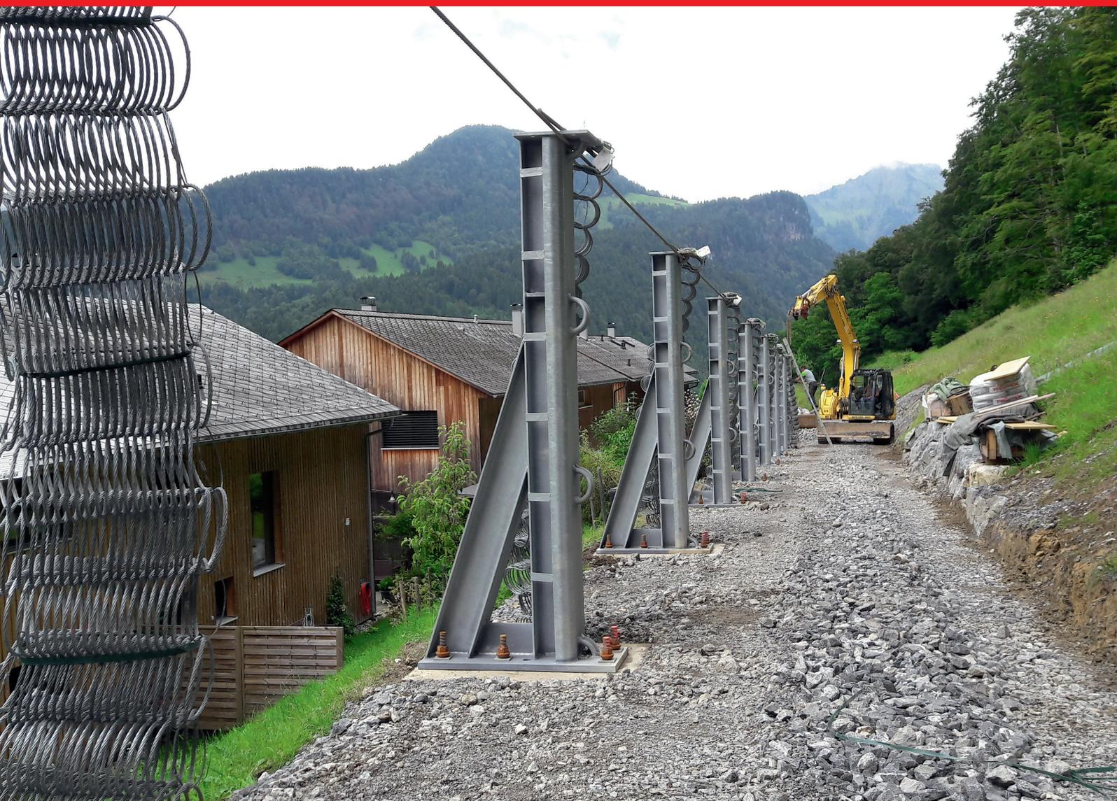
The delta-frame Debris Catcher is a post-supported flexible-net barrier that can be installed in wide channels or along open slopes. The retention capacity of this system is controlled by the gradient of the slope and the height of the posts. An endlessly long system can be designed whereby independent sections are defined by internal anchoring of bearing ropes.
