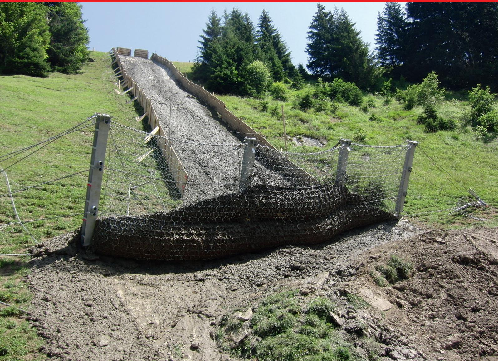
Shallow landslide barriers are systems evolved from rockfall catchment fences. As they are a post-supported system, they can be used in wide channels or along open slopes. These systems are especially suitable for the installation sites having difficult terrain.
